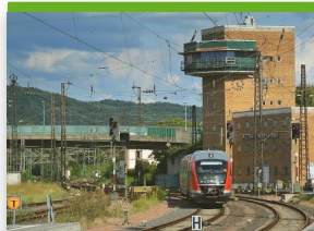
Railway control centers
