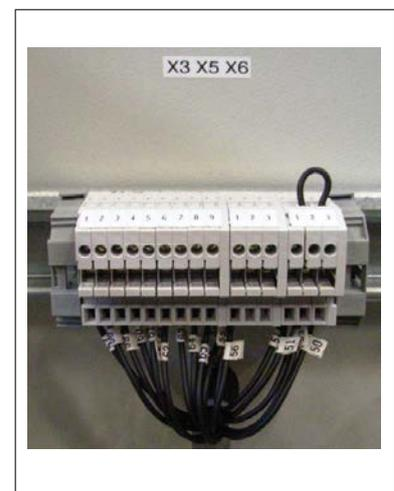
When an alarm occurs, the X3 relay contacts are de-energized and switch.
