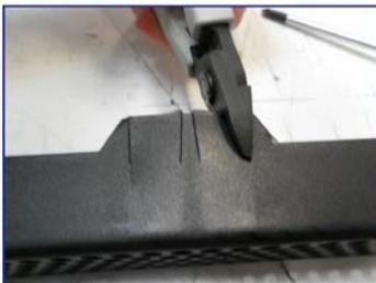
**Cut holes to allow cable access**
