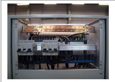
The standard AC output distribution unit is designed with a 35 mm DIN rail, Multi Clip termination board and N/PE copper terminal bars, and built as a part of the cabinet.
